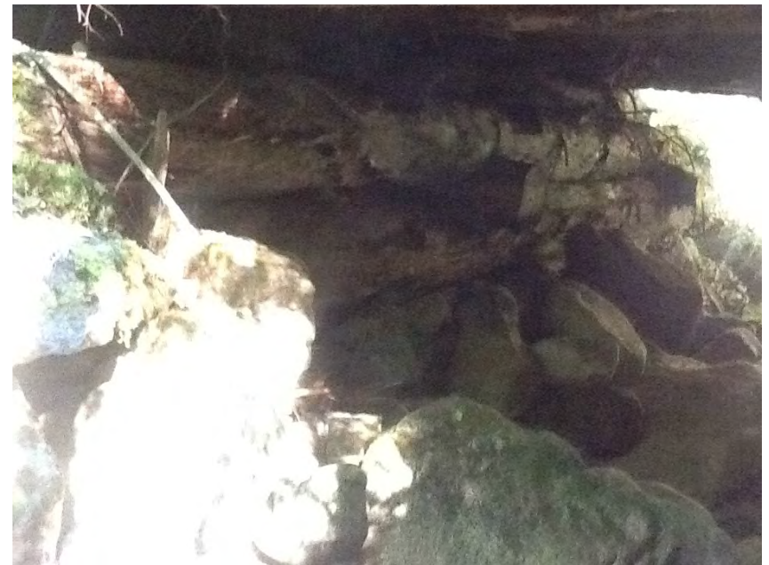
Left Bank Abutment when facing downstream
