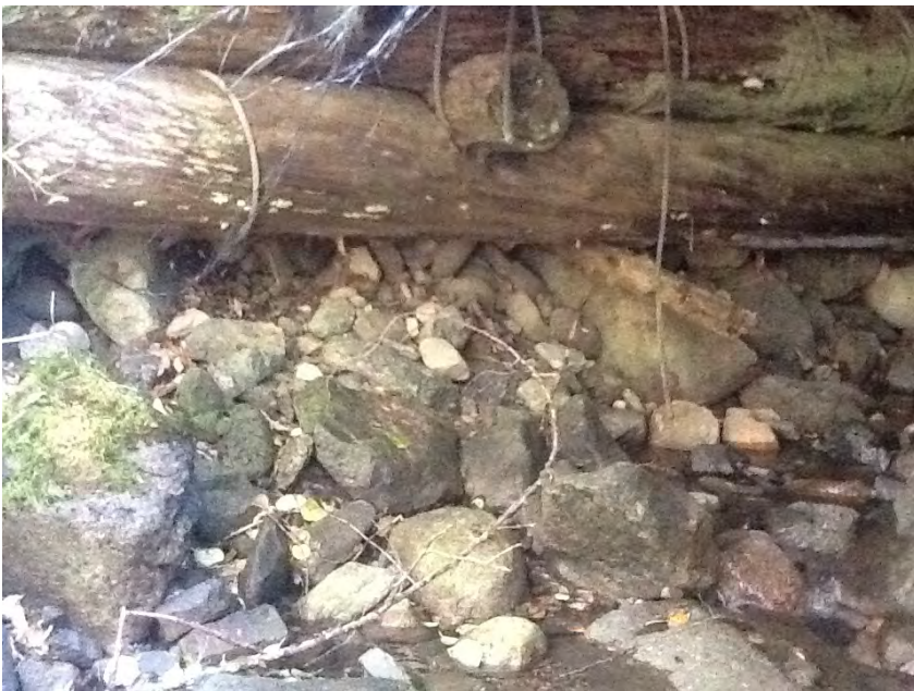
Right Bank Abutment when facing downstream
