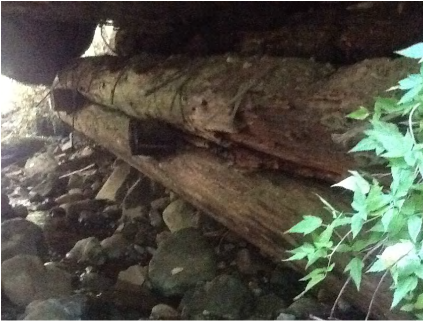
Right Bank Abutment when facing downstream
